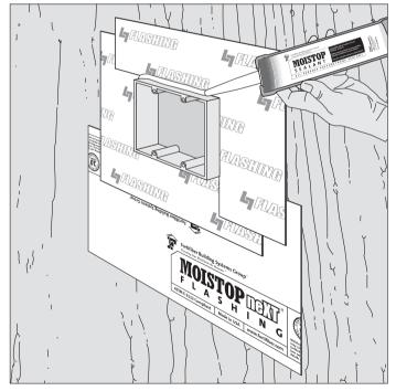
Apply final %" bead of **Moistop Sealant** and tool it around utility box.
