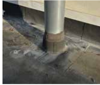
Pipe penetration/cracking
