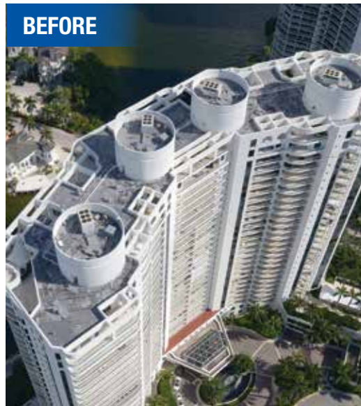
Photos courtesy of Florida Quality Roofing
