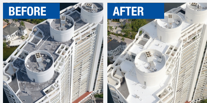
Photos courtesy of Florida Quality Roofing
