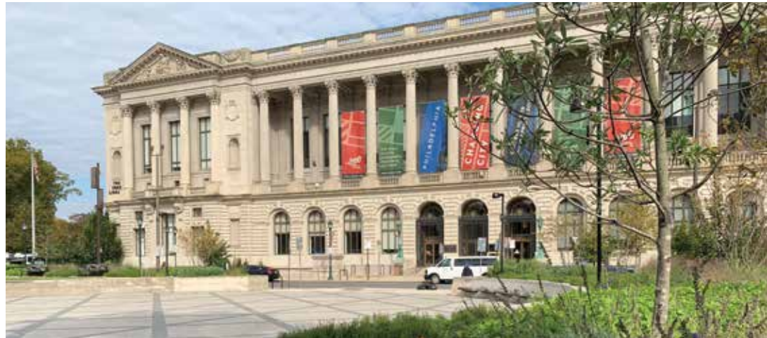
Green Roof and Plaza, Philadelphia, PA
