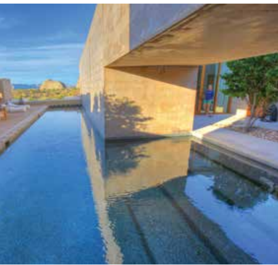
Water Containment System, UT
