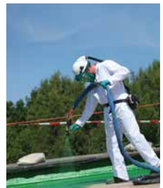
Installation of Prodeq FX400 membrane
