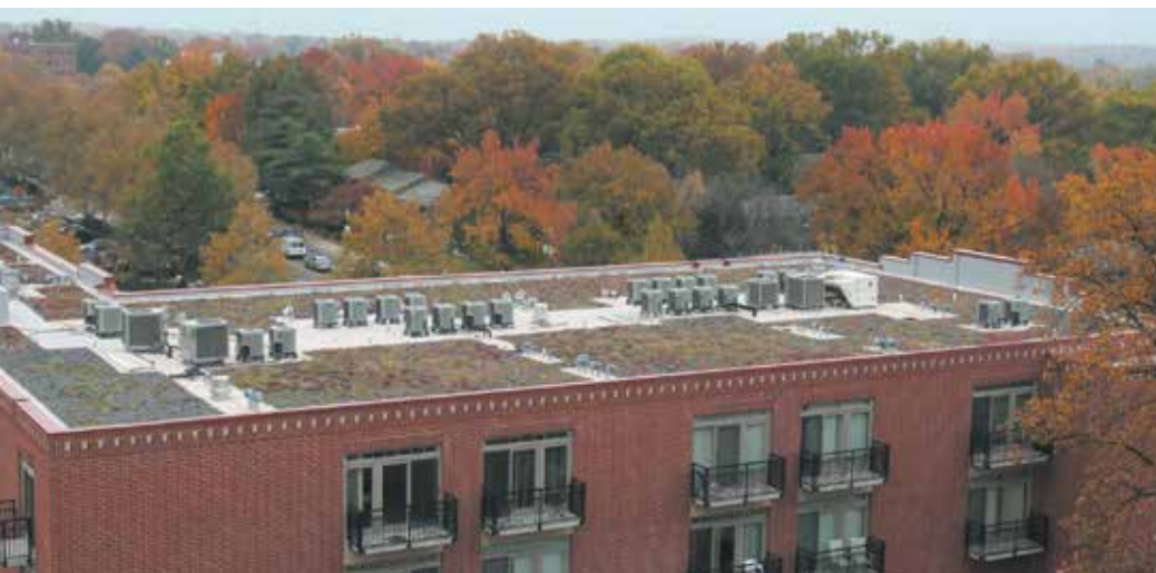
Green Roof, Falls Church, VA
